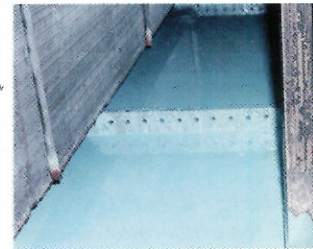
A Rusted Pan treated with PANCRETE®
